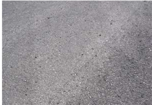
Figure 13 Low Severity Raveling
